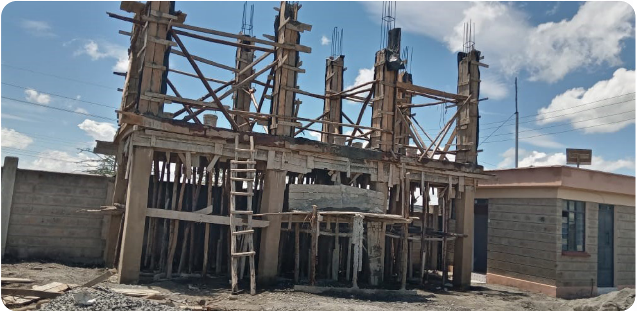
Ongoing Water Tower Construction in one of our Projects.
